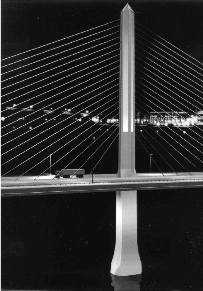
PHOTO 5.1 A rendering of the new Maumee River Bridge, Toledo, Ohio. This cable-stayed bridge spans the Maumee River in downtown Toledo as a monument icon for the city. The design includes single pylon, single plane of stays, and a main span with a horizontal clearance of 612 ft in both directions. The main pylon is clad on four of its eight sides with a glass curtain wall system, symbolizing the glass industry and heritage of Toledo. This glass prismatic system and stainless steel clad cables create a sleek and industrial look during the day. At night, the glass becomes very dynamic with the use of LED arrays back-lighting the window wall. Owner: Ohio Department of Transportation (courtesy of the Designer, Figg Engineering Group, Linda Figg, President, Tallahassee, Florida).
