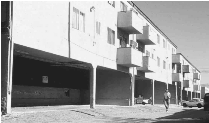
FIGURE 7.7 Typical soft story “tuck-under” parking, with apartments above (courtesy of EQE International).
