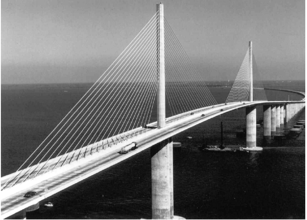
PHOTO 5.7 Sunshine Skyway Bridge, Tampa, Florida. Designed by Figg and Muller Engineers, Inc. The bridge has a 1200 ft cable-stayed main span with a single pylon, 175 ft vertical clearance, a total length of 21,878 ft and twin 40-ft roadways (courtesy Portland Cement Association).
