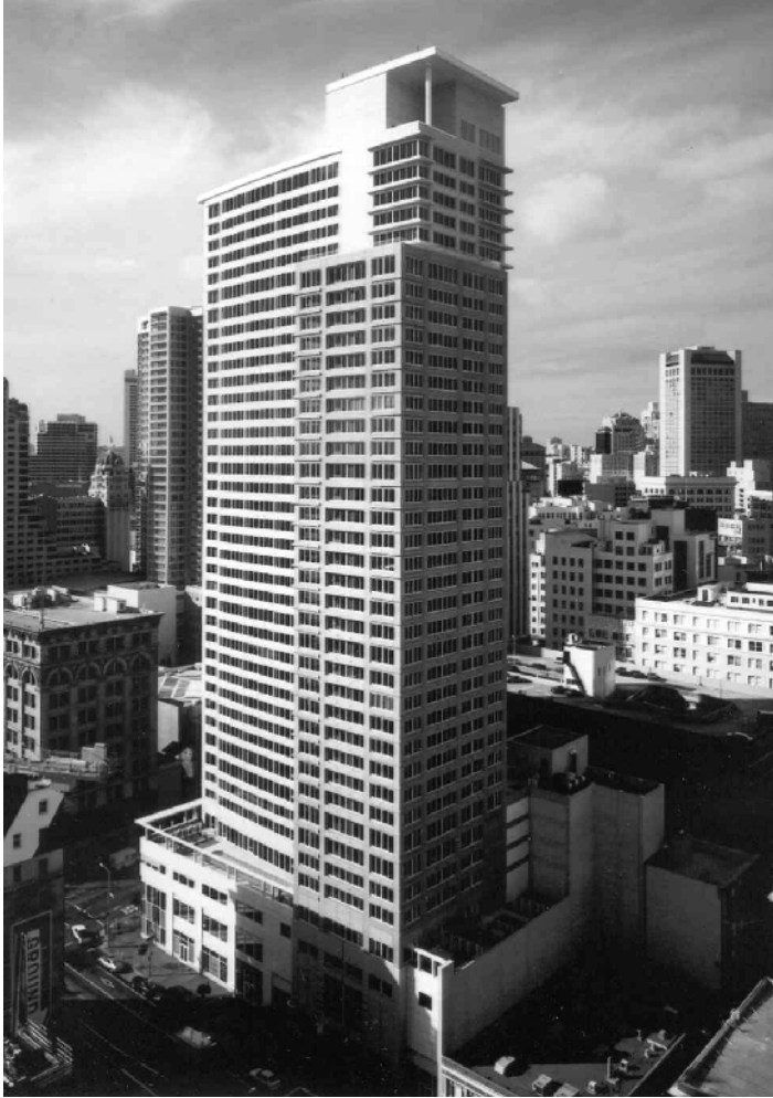
PHOTO 5.4 Paramount Apartments, San Francisco, CA: completed in 2002, it is the first hybrid precast prestressed concrete moment-resistant 39 floor high-rise frame building in a high seismicity zone. Based on tests of large-scale prototype of the moment-resisting connections, it was determined that the performance of the system was superior to cast-in-place concrete, both in cracking behavior and ductility. Hence, as a system, this new development succeeds in enhancing the performance of high-rise buildings and bridges in high seismicity earthquake zones. Since completion of this structure, several other buildings in California have been completed using the same principles (courtesy Charles Pankow Ltd, Design/Build contractors. Structural Engineers: Robert Englekirk Inc.).
